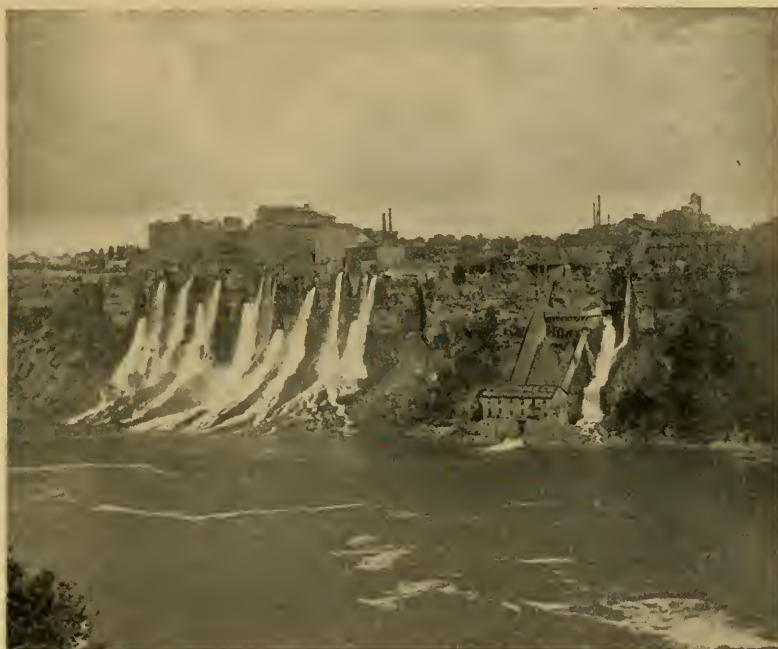
THE AMERICAN BANK BELOW THE STEEL ARCH BRIDGE, SHOWING THE WASTE OF WATER AND POWER FROM THE SPILLWAYS AND TAIL-RACES OF THE FACTORIES.
